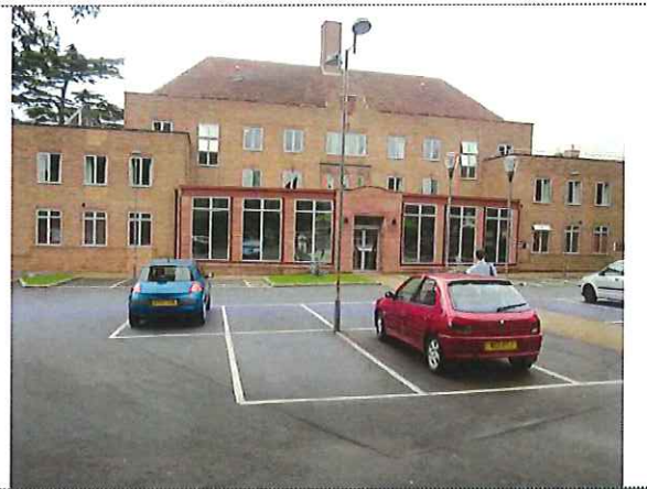
Parking to the front of Gardner Hall entrance
