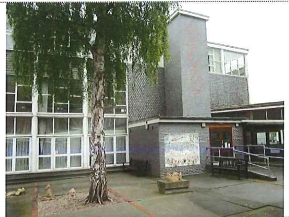
Entrance into Sports Hall from Main Building
