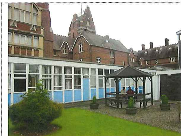
Rear single storey annex to Main Building
