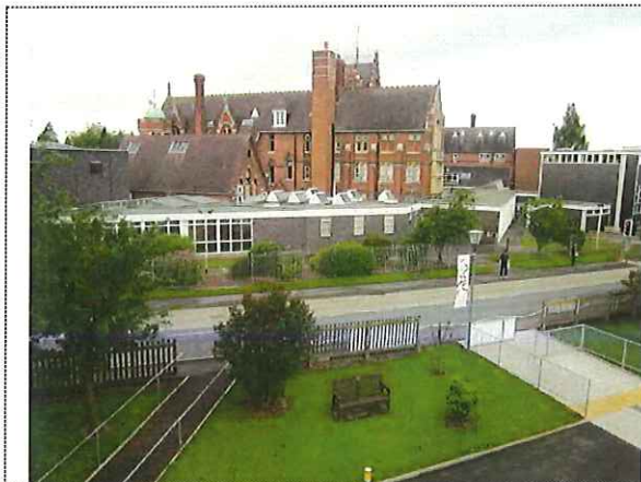
East wing from across Venns Lane – Music block mid ground Sports hall RHS
