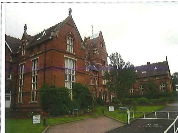
West wing of southern frontage (main entrance)
